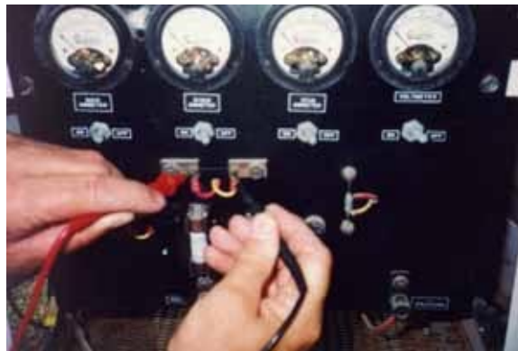
Figure 1.5. Measuring Rectifier Output Current.
