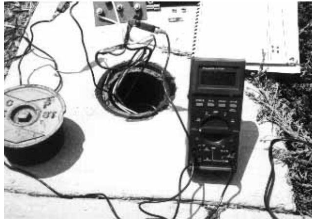
Figure 1.7. Measuring Output Current of Galvanic Anode.
