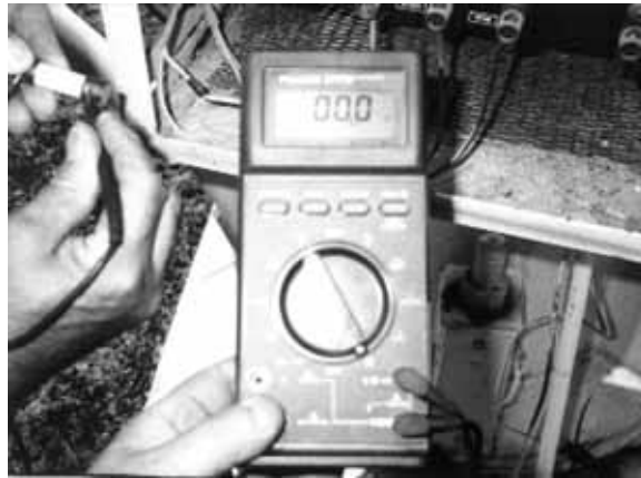
Figure 2.3. Verifying Continuity of Fuse.
